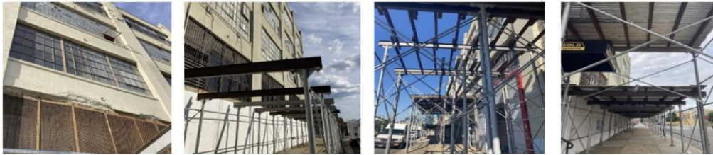
Figure 2: Different phases of sidewalk shed erection
