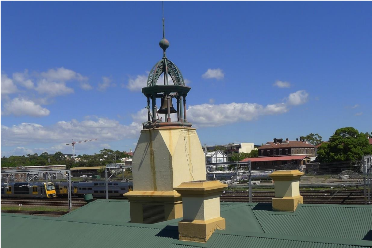
Figure 2. The belfry and tower prior to conservation (The author 2014)
