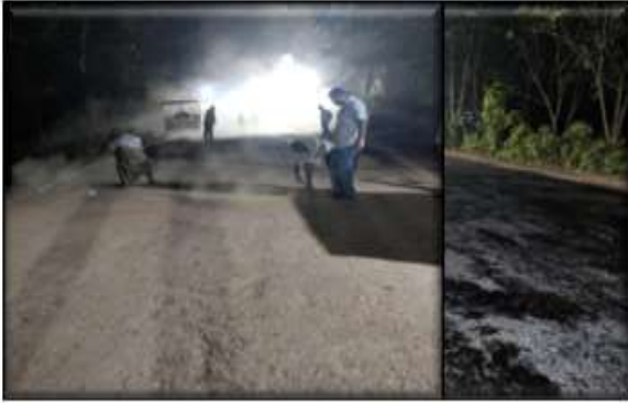
Cleaning and applying bitumen emulsion
