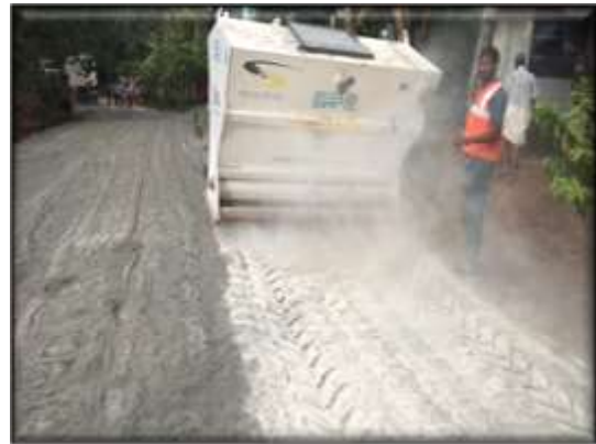
StabilRoad Spreading
