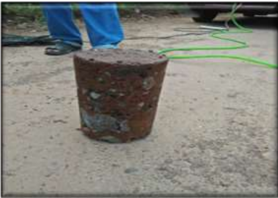
Extracted core From Stabilized Base
