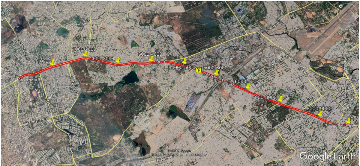
Fig.3.3 Satellite view of 10 km road stretch in Hyderabad
